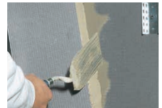
The Austrotherm UNIPLATTE® panels can be fitted immediately. This ensures a right angle.
