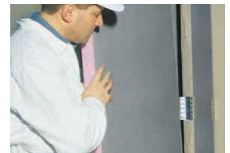
One Austrotherm UNIPLATTE® already fits nicely into the other.
