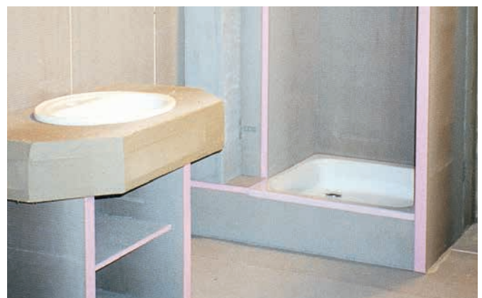
Separating walls for building shower cubicles provide the best substrate for ceramic tiling.
