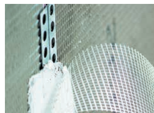
Panel joints are closed off using glass fibre fabric strips.
