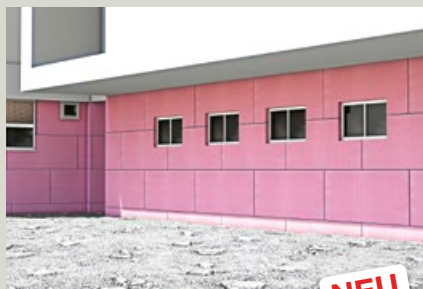
Austrotherm XPS® PLUS P \lambda_D = 0,032 \text{ W/(mK)}
