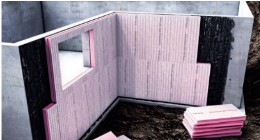
▶ Exterior cellar wall
