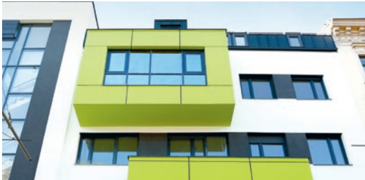
Façade insulating board with Austrotherm TOP coating compound.
